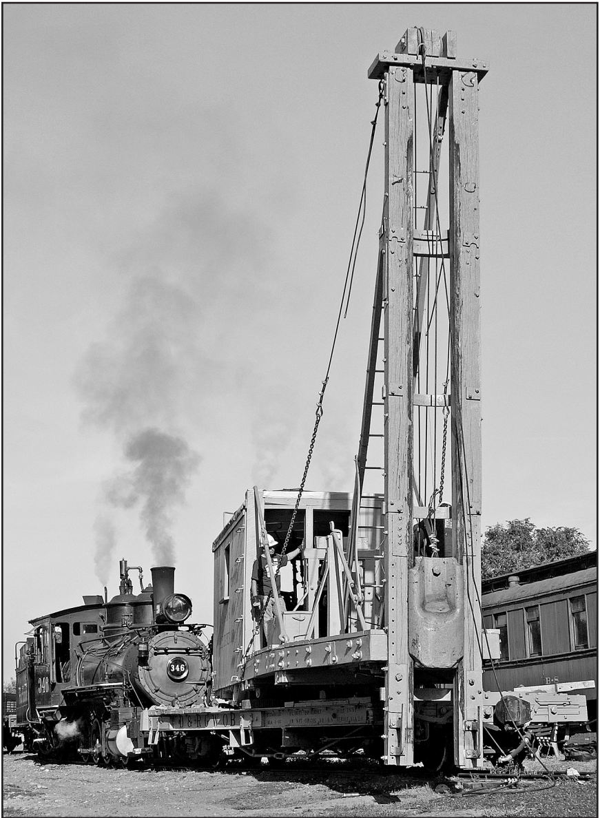
Rio Grande pile driver OB was powered by engine #346 on its first demonstration day at the CRRM on September 17, 2009. – Photo © 2009 Dave Schaaf.
